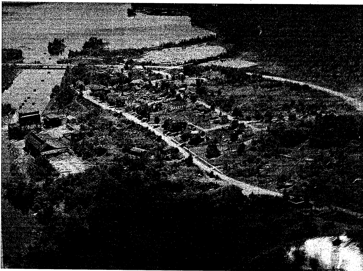
Aerial photograph of Piercefield, looking south, dated to the 1950s, judging from the automobiles. Remains of the International Paper mill and log boom anchors in the Raquette are still visible at left. The highway bridge to Tupper Lake is upper left. Photo courtesy Piercefield Museum.
